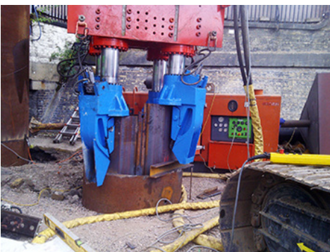
Crane suspended vibro installing Ø1.520 (2off)
