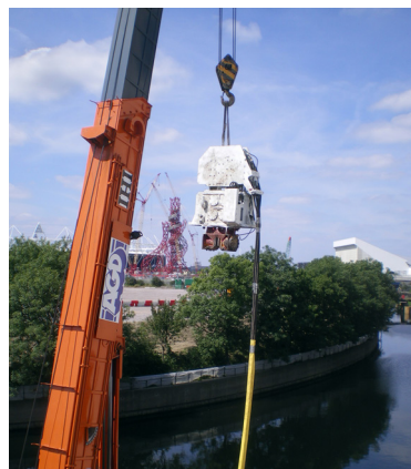
Crane suspended vibro installing AU25 with single clamp head
