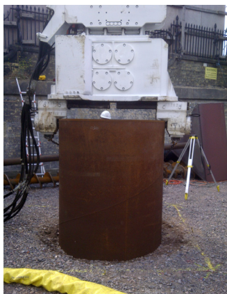
Crane suspended vibro installing Ø1.520 (2off)
