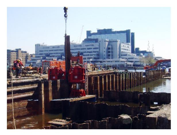
Contractor Dawson-WAM selected the X1000 pile extractor to remove more than 1500 sheet piles at the prestigious Canary Wharf development in central London. The 22m (72') long Corus LX25 piles had been driven as pairs to refusal with a 7t hydraulic drop hammer some 6 years earlier. Extraction had to be undertaken safely, without vibration and at low noise levels.
