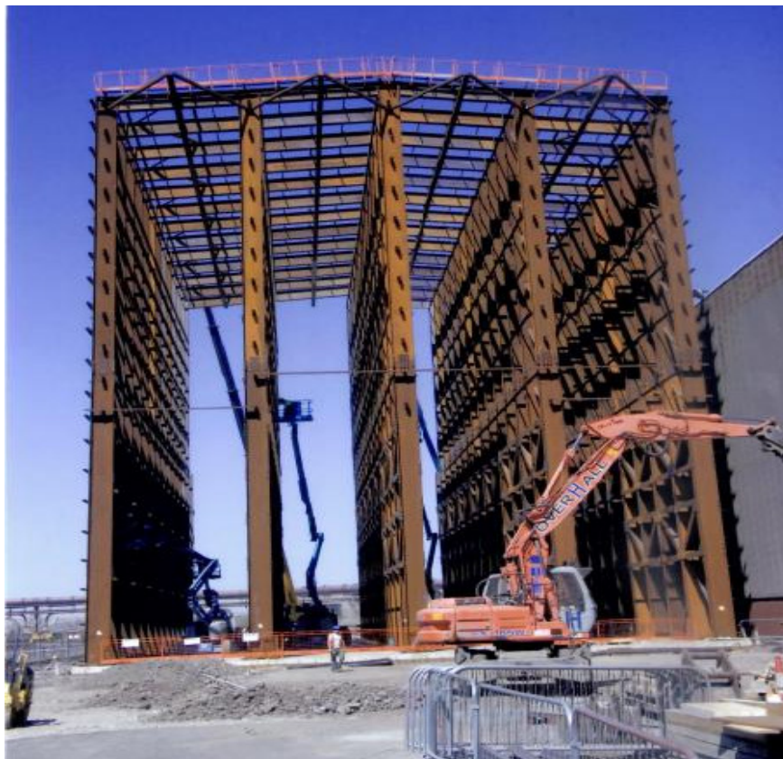
The ADC structure 159m long, 25.7m wide and 30m high
