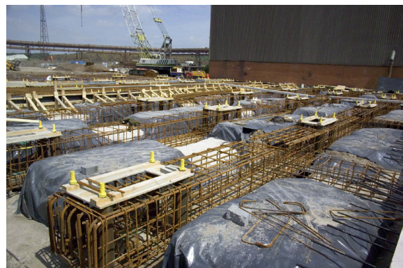
Pile caps and holding down bolts
