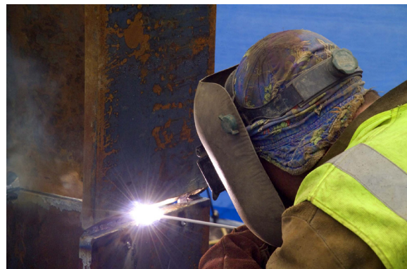
Splice welding the piles together
