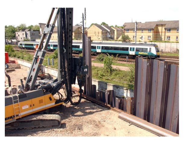
Major UK contractor Kier London, in onjunction with Corus Hydrobarrier, used the Dawson Contract Piling Ltd, to form the watertight retaining walls of a new rectangular basement. The basement formed part of a new £26m development. This contract was to be the first time that the new "wide" U profile sheets were to be installed using hydraulic pressing.
