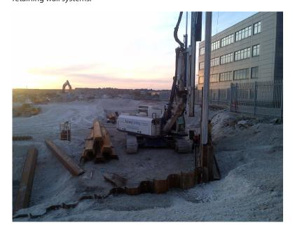
An independent Noise & Vibration Assessment was undertaken to establish the constraints on installation methods, taking into account the existing warehouse unites approximately 15m to 20m from the pile line. Fussey Piling proposed the use of one of their Bauer RTG16T telescopic leader rigs, which vibrated the piles to the required levels within a 2 week programme, using a high frequency variable moment vibrator.
