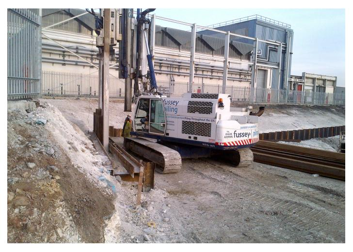
Client **Bowmer & Kirkland** Scope Permanent sheet piled retaining wall with heights up to 5.0m Contractor **Fussey Piling Limited Piles** Arcelor Mittal PU18-1mm, PU22-1mm, Location Basingstoke, UK PU22+1mm and PU28-1mm in lengths October 2012 Date 7.0m to 12.0m (Grade \$355GP) £160k approx. Value **Ground Conditions** Structureless Chalk (White Chalk Sub-**Duration** 2 weeks group)
