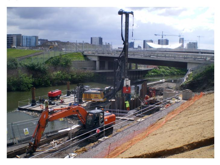
Main contractor Bam Nuttall selected Dawson Contract Piling to install 5m temp and 10m permanent sheet piles. The permanent piles were set to level using a 2 cylinder silent and vibration less system, to form a retaining wall along the river on the Olympic site. Work was carried out on a 20m x 20m floating pontoon using a LRB125 piling with a Ø400 auger / resonance free vibrator/ 2 cylinder push pull system and was completed safely and on time to the clients requirements.
