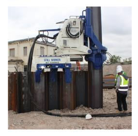
A hard band of Limestone is present within the Lambeth Group beneath much of the Greenwich peninsula, at varying depths associated with the many geological faults in the vicinity. Early engagement ensured that the risk of encountering this band was explored with additional deep boreholes undertaken in advance of the detailed design. The toes of the sheet piles were proven to reach only into the River Terrace Gravels, which sit above the Lambeth Group.
